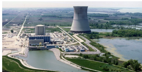
Davis-Besse nuclear plant | FirstEnergy
